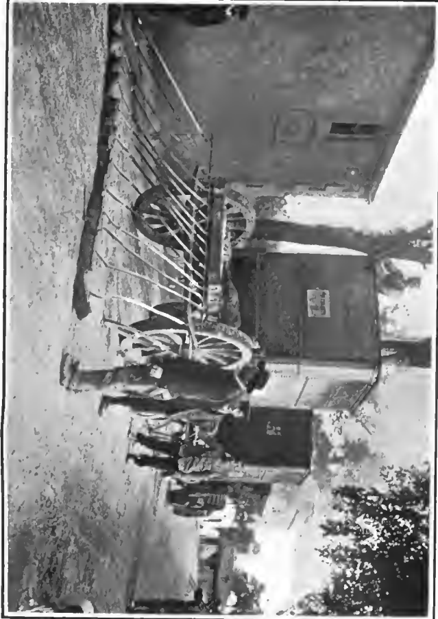
Sprinkling the Course with Tarry Fluid, which Brushes Distribute Evenly. VIEWS ALONG THE AUVERGNE CIRCUIT IN FRANCE, SHOWING INTERESTING FEATURES OF THE PREPARATIONS FOR THE INTERNATIONAL GORDON BENNETT RACE. TO BE HELD JULY 5.
